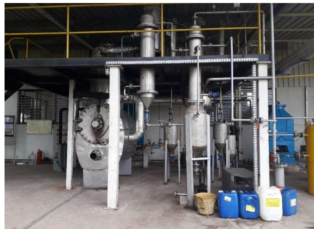
Use of Plastic fuel for burners and material handling equipment
